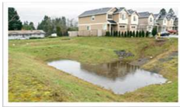
Infiltration basin – Bazen za infiltraciju
